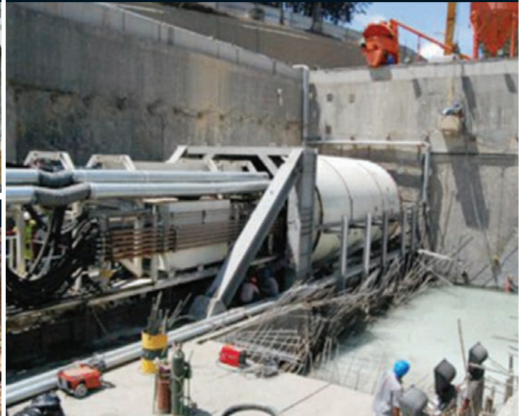
Tunnel Boring Machine
