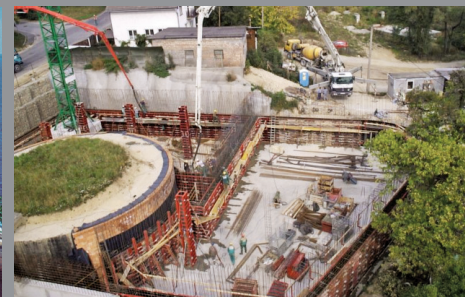
Koliba Water Reservoir, Bratislava
