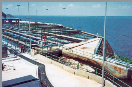
Ponta Do Ismael Water Treatment Plant, Brazil
